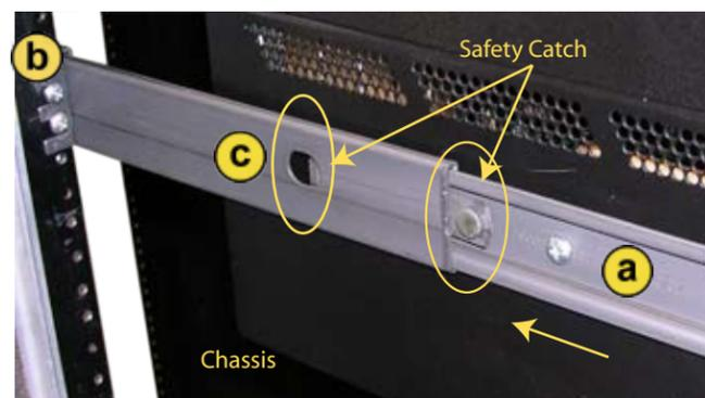
Next, press on the safety catch on slide piece **a** and continue to push until it stops again. Press on the safety catch again to allow the chassis to slide all the way into the rack.
